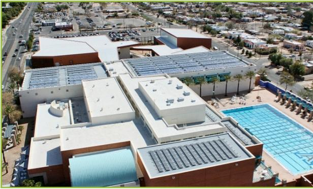
Solar generated hot water is utilized to heat the swimming pool at the Campus Rec Center
