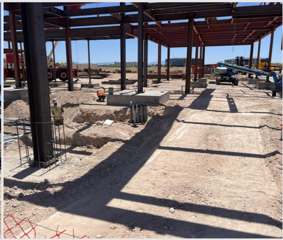
View of level 1 from the Northwest corner
