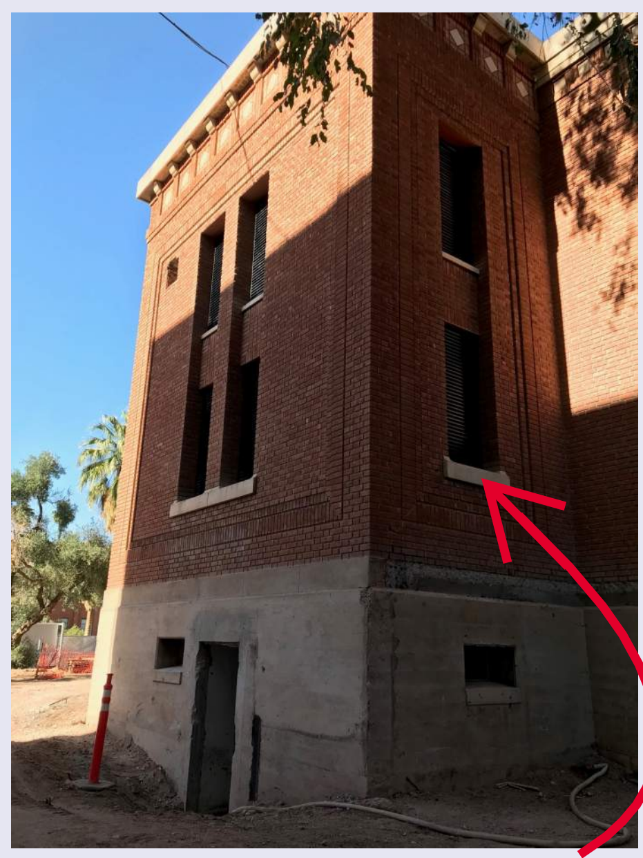
The mechanical team has installed new louvers in the windows in the northwest corner. They will provide the air-intake for the entire building!
