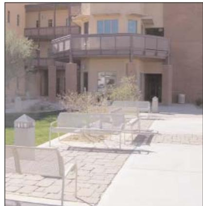
*Unit pavers with standard gray concrete pedestrian pavement (The University of Arizona)*
