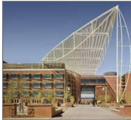
Thomas W. Keating Bioresearch Building
