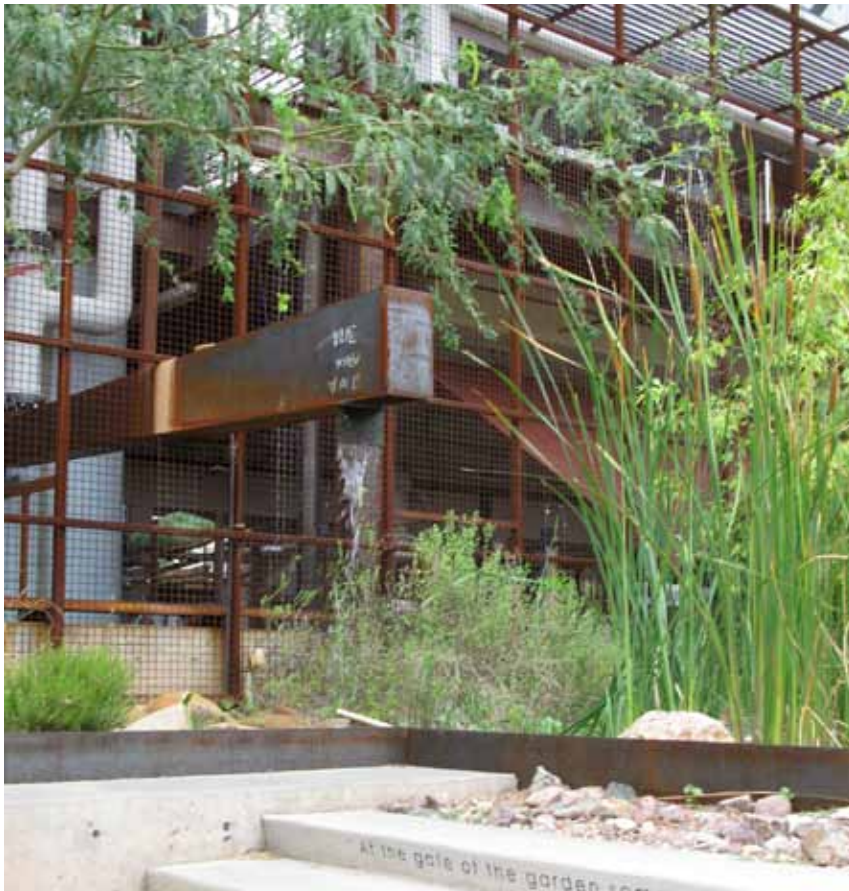
CALA building addition green wall (behind) and the multi-habitat bioswale and demonstration garden with recycled rain water (in front).
